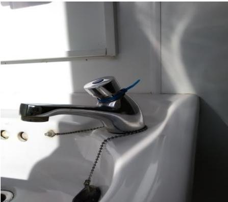
*The simple cable tie reduces water consumption on our site in Welling*
